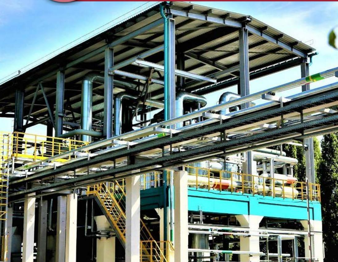
**Vacuum evaporation unit for VOCs**
